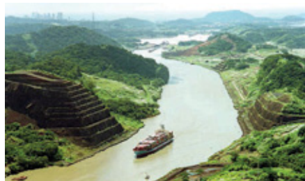
Gaillard Cut, Panama Canal
